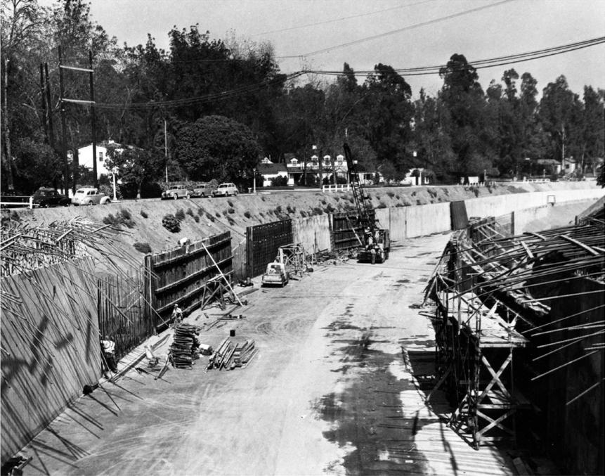
FIGURE 36. The Los Angeles River being prepared for concrete.
