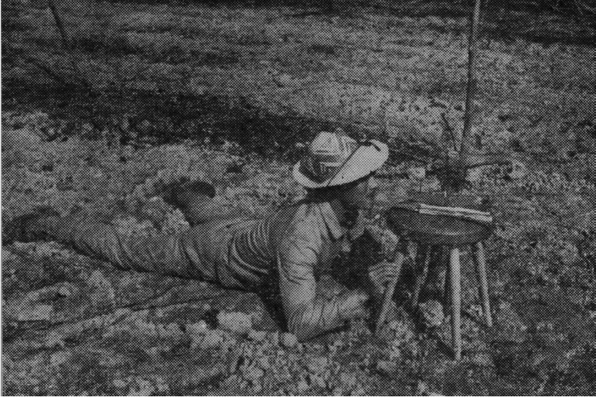
FIGURE 28. “Straw Hat Diplomats” exemplified the ingenuity of Taiwanese technicians in conditions where state-of-the-art tools were too expensive or difficult to acquire. The one pictured here was a member of the Taiwanese team in Liberia shown with a “makeshift level” on an ordinary stool. Wang, “Straw Hat Diplomats.”
