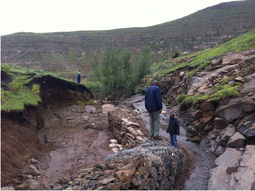
FIGURE 4. Collapsed streambank after a storm in the village of Khahleti. Photo by author.
