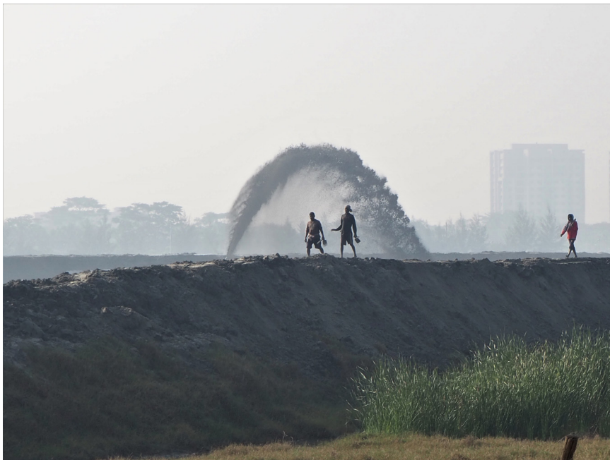
FIGURE 25. Dredge discharge pool on the banks of Mongla River.
