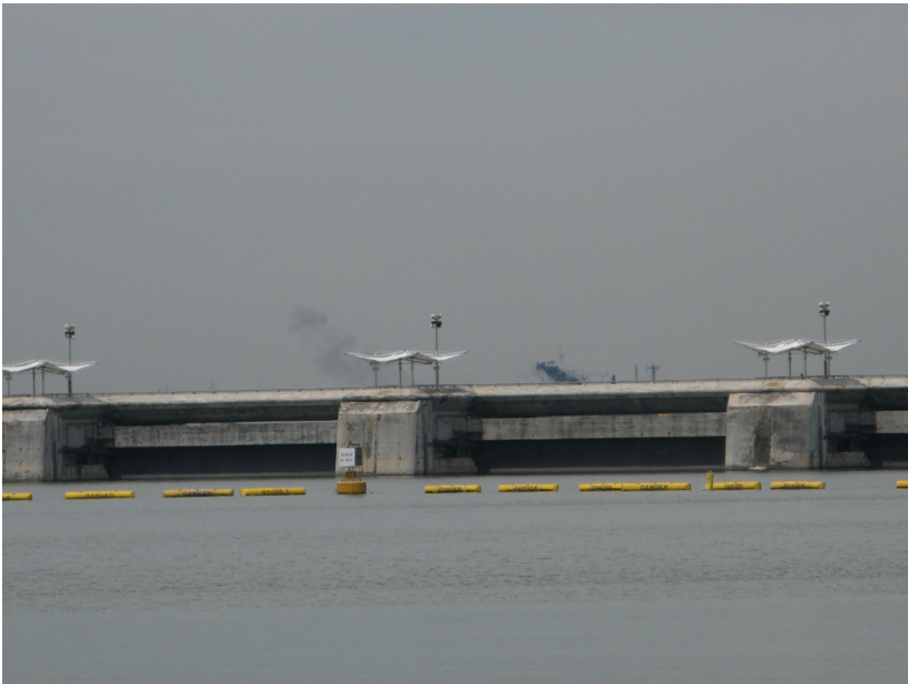
FIGURE 10.5B. The Marine Bay Barrage regulates the island's floods and the freshwater catchment system.
